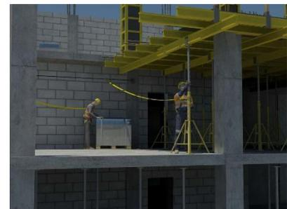
Restraint systems are made up of a harness that is connected to an anchor point or static line using a lanyard. The anchor point should be designed for fall-arrest loading.
