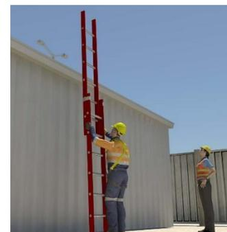
Depending on the type of work you are doing, you might need to use a fall prevention system that is connected to a ladder.
