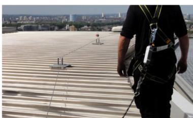
Static lines are horizontal lines that a lanyard can be attached to
