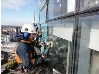
Industrial rope access systems allow workers to be suspended from vertical ropes to access the work area which could be the side of a building or down in an area that can only be accessed through an opening up high (such as a tank or silo).
