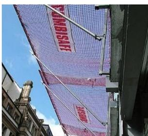
Catch platforms and safety nets are short term structures that are installed below a work area to catch a worker if they fall or to catch falling objects.
